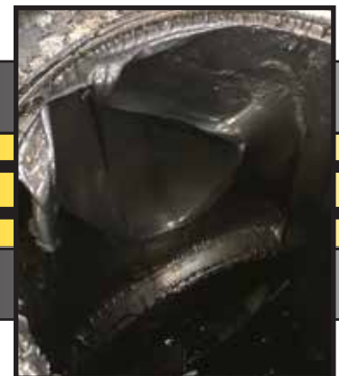
Valve Cavity after 52 stage job
