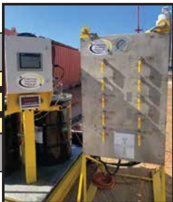
Grease Purge System
